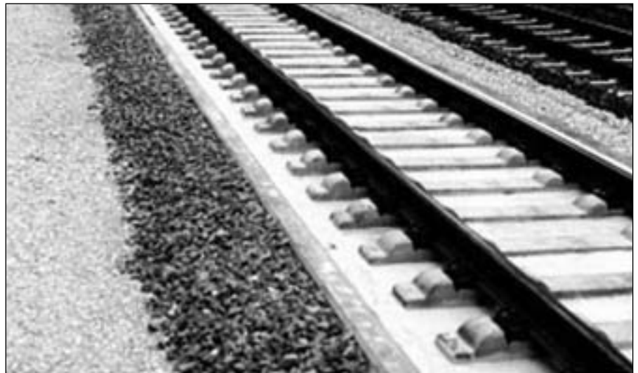
Concrete slabtrack would dramatically reduce rail maintenance.
