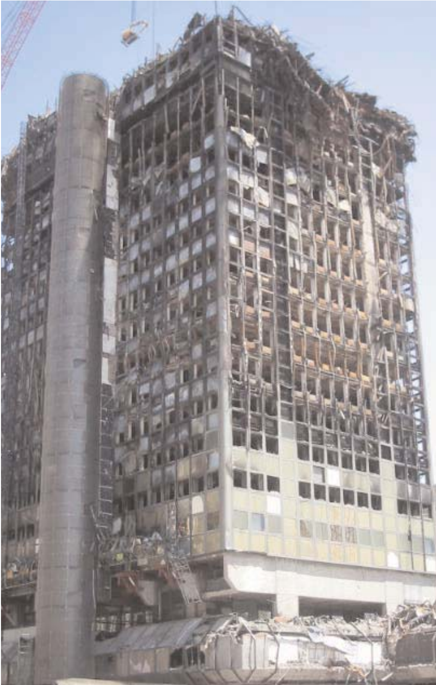
Windsor Torre during deconstruction.
