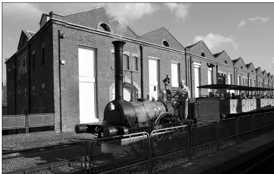
Replica locomotive, Planet, steaming past the Grade I listed building.
