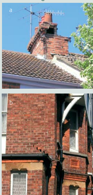
Damage from the 2007 Folkestone earthquake: (a) Damage to a chimney and (b) structural damage, to Victorian masonry houses in Folkestone.
