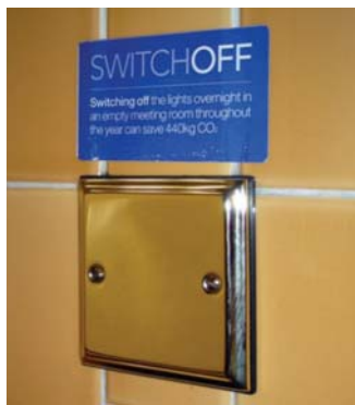
Ambiguous controls create confusion and can lead to users distrusting the system or simply ignoring subsequent useful information or control signals.
