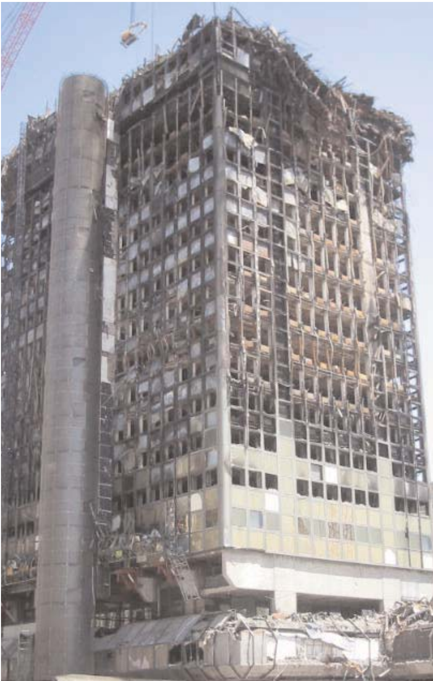
Windsor Torre during deconstruction.
