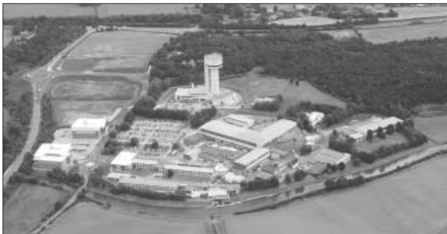
The CCLRC Daresbury Laboratory showing the new Daresbury Innovation Centre and the Cockcroft Centre to the left of the site. The surrounding land has potential for further expansion.
