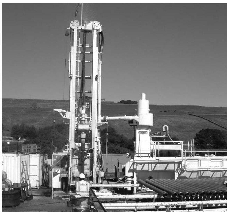
Drilling the borehole into the Weardale granite in County Durham
