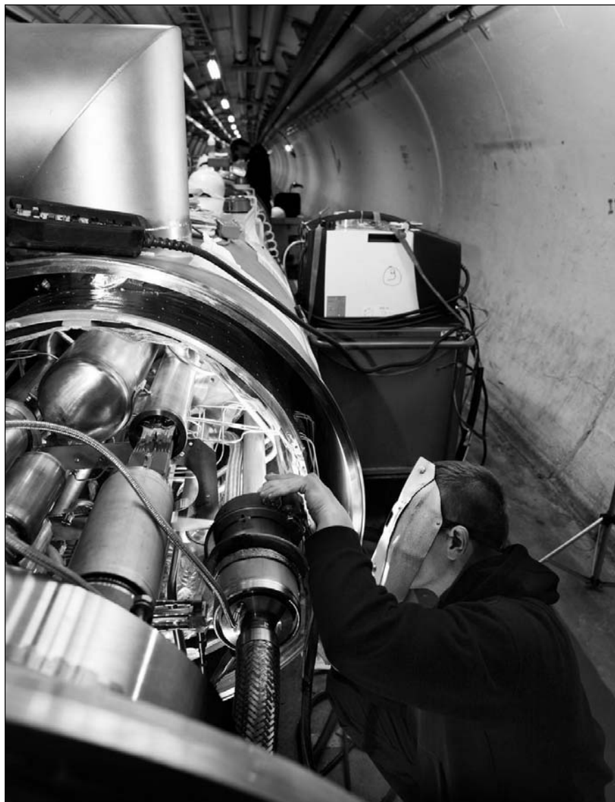
A welder closing one of the interconnects between LHC magnets
