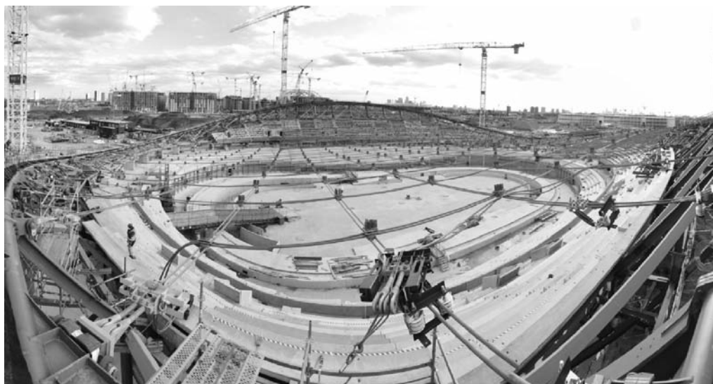
Cablenet roof design at the Velodrome
