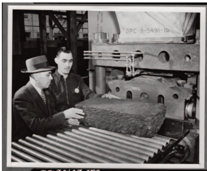
Fig 2. Synthetic rubber production, circa 1940. Rubber was a vital material for vehicles and clothing, and mass production of synthetic rubber became necessary when natural rubber supplies were cut off in 1942. Businesses agreed to share patents and scientific information to solve the rubber crisis. By 1944, 51 new production plants were producing 800,000 tonnes annually. 2 (Image: Library of Congress, LC-USW33-028402-C.)
