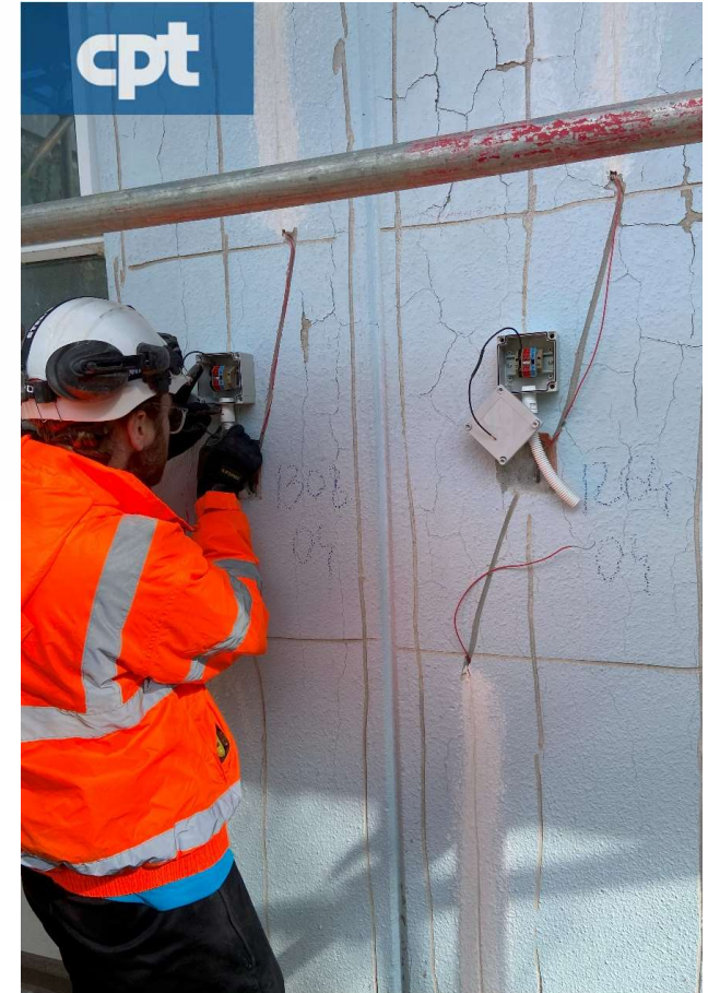
Installation of RAACGuard Anodes
