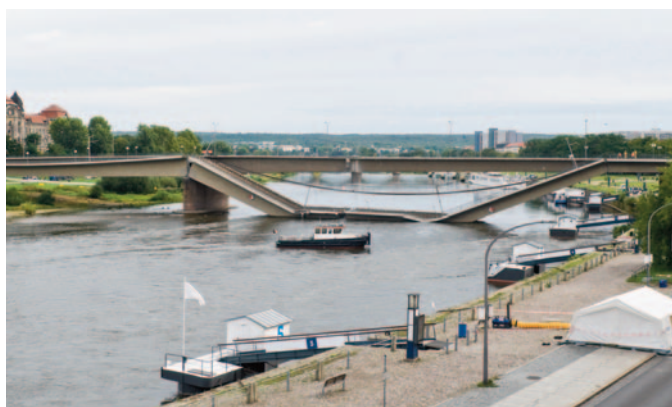
Collapse of the Carola Bridge on the River Elbe in Dresden, Germany, in September 2024. There were no fatalities but significant disruption occurred, including the loss of hot water supply for the entire city and halting of shipping on the river. A formal investigation is ongoing but local authorities have stated that corrosion of steel reinforcement due to ingress of salt is likely to have been the cause of the failure.
