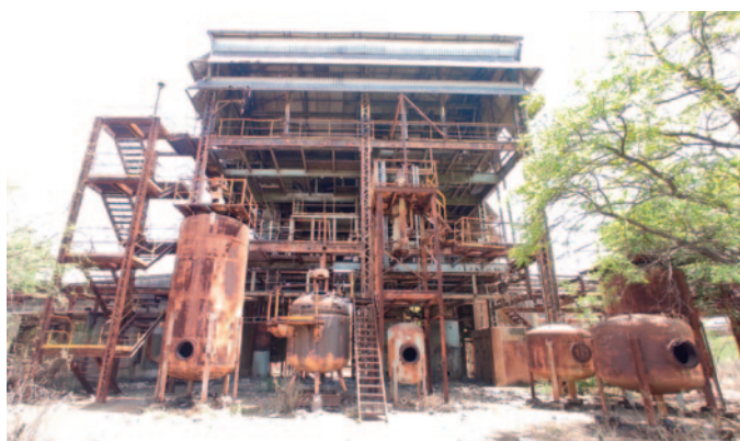
Site of the Union Carbide disaster in Bhopal, India, considered by many to be the world's worst ever industrial tragedy. Corrosion was a significant contributing factor to an explosion at this insecticide plant in October 1984, which led to the release of a large cloud of toxic gas. The final death toll was estimated to be between 15,000 and 20,000.
